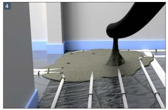
Apply the screed layer referring to the screed manufacturers instructions for mixing, drying and curing information.
