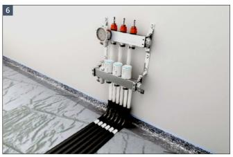
Install pipe conduit or lagging over the service pipes as this will insulate the pipes and alleviate any hotspots.
