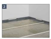
Lay a damp proof membrane over the subfloor to prevent water ingress.
